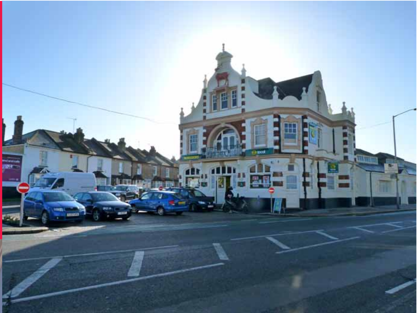
Front elevation and customer car park from Brighton Road
